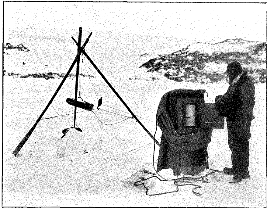
FIG. 1.—BAGE AND THE TIDE GAUGE.
