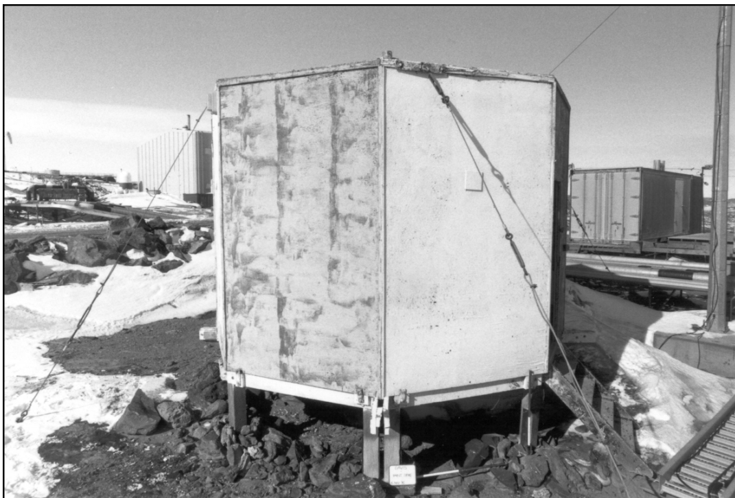
Paint Store (View of northern side)
