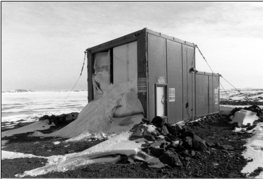
Old Balloon Hut (View of northern and western sides)
