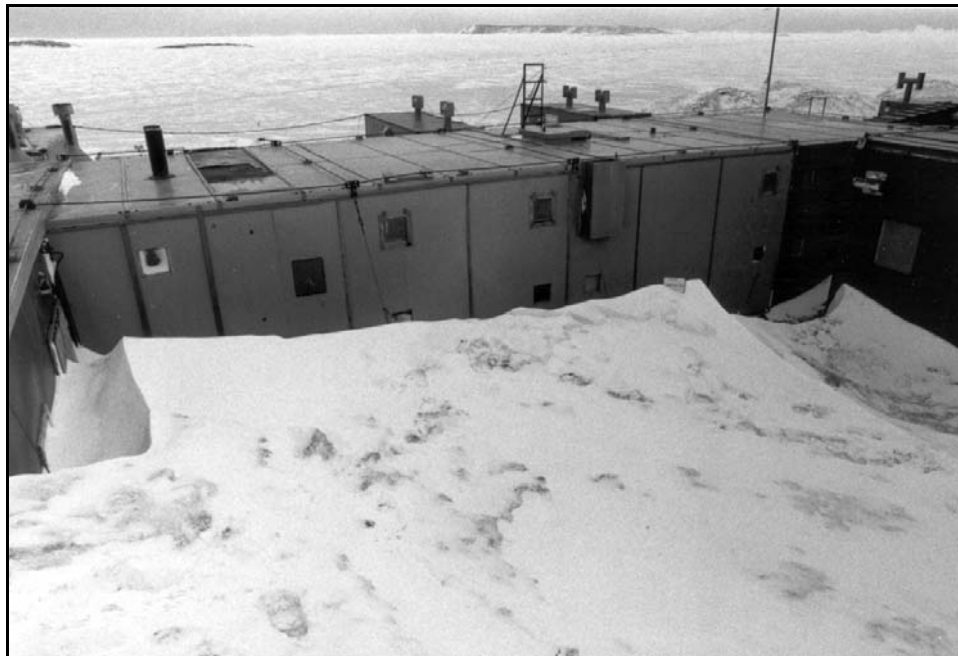
Sleeping Hut (View of eastern side)
