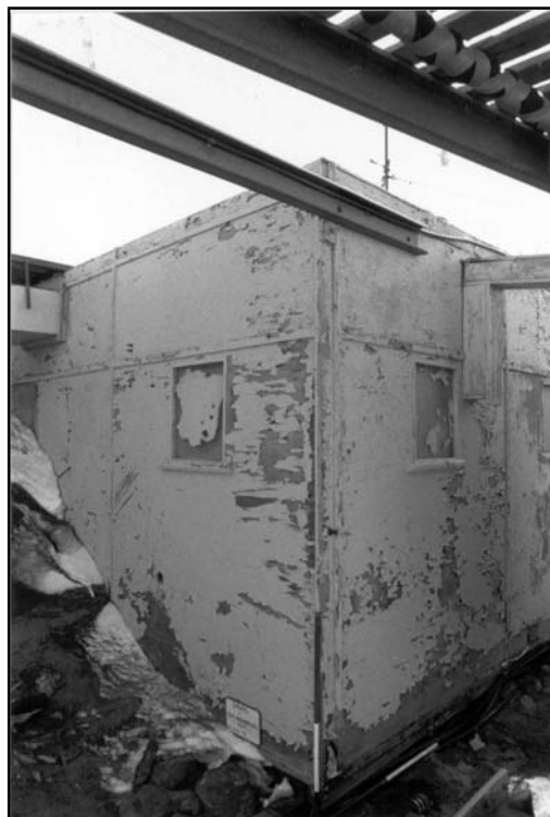
Old Recreation Hut (View of southeast corner)
