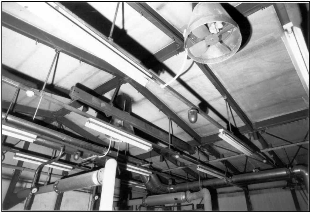
Emergency Powerhouse (Ceiling detail)
