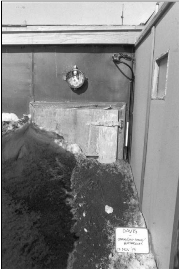
Office/Cold Porch/Bathroom (North wall detail)
