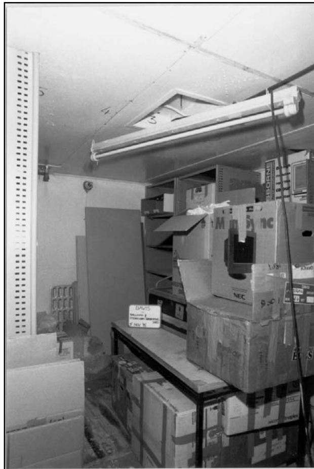
Old Balloon Hut (Interior view, Eastern Room)
