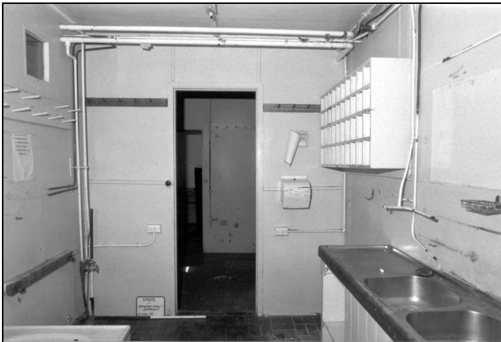
Office/Cold Porch/Bathroom (Interior view of Bathroom, looking east)
