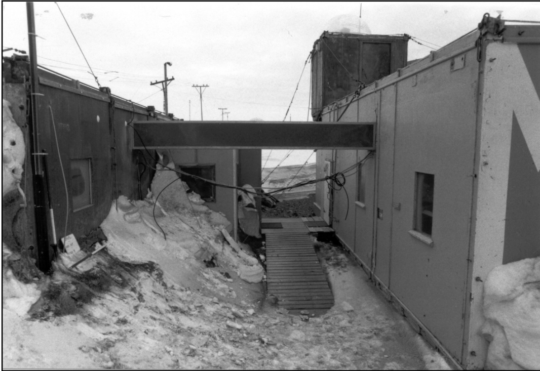
Link between Met Office (right) and Radio Hut (left)
