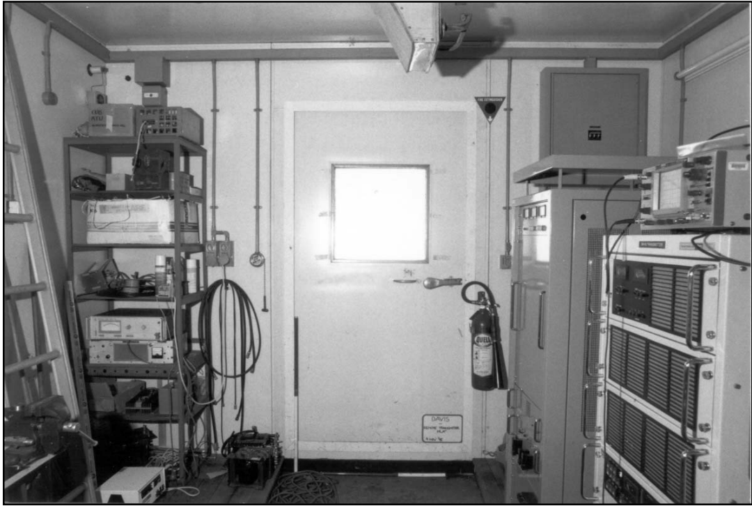
Remote Transmitter Hut (Interior view looking south)
