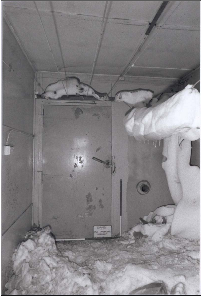
Old Carpenter's Workshop (Interior view of Original Room, south wall)
