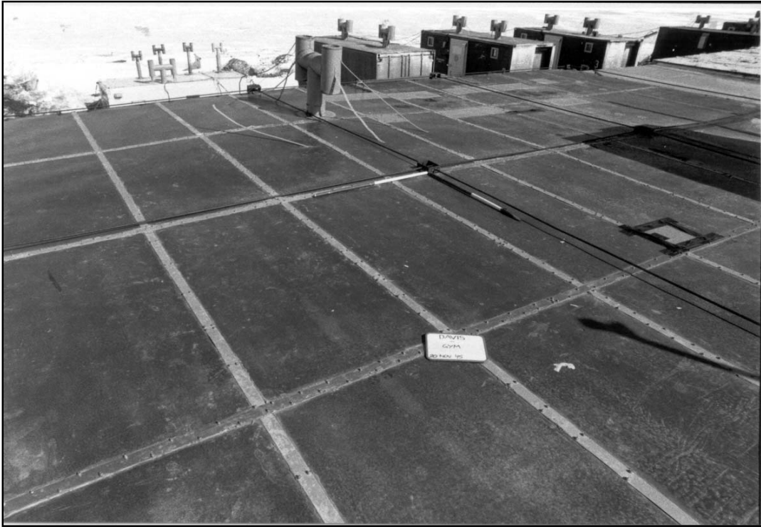
Gymnasium (Roof detail)
