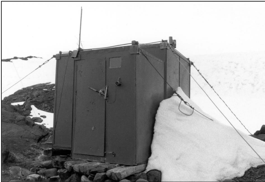
Old Platcha Hut (View of Cold Porch)
