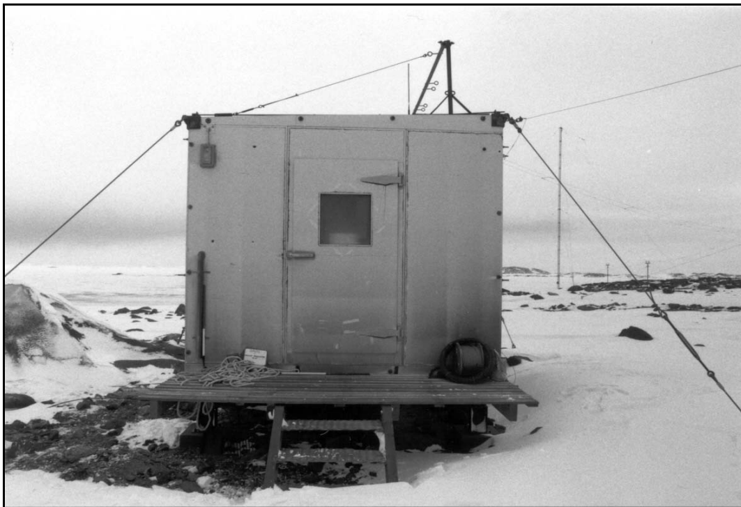
Remote Transmitter Hut (View of southern side)
