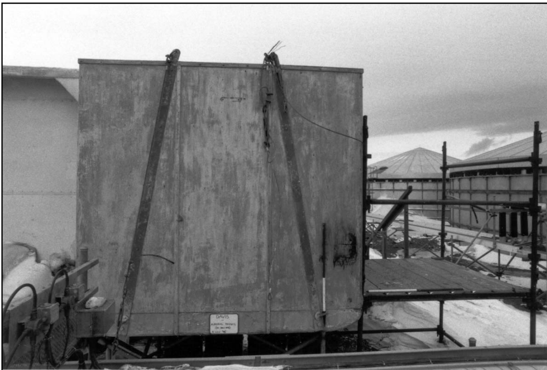
Emergency Radio Transmitter (View of western side)
