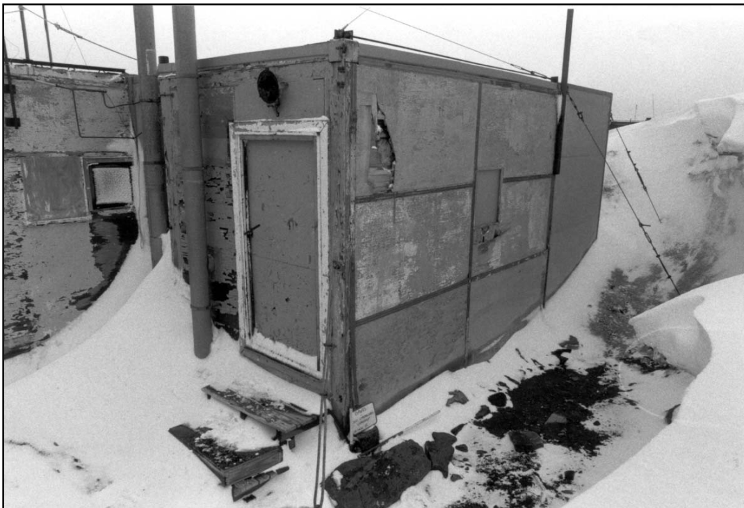
Old Carpenter's Workshop (View of eastern and southern walls)
