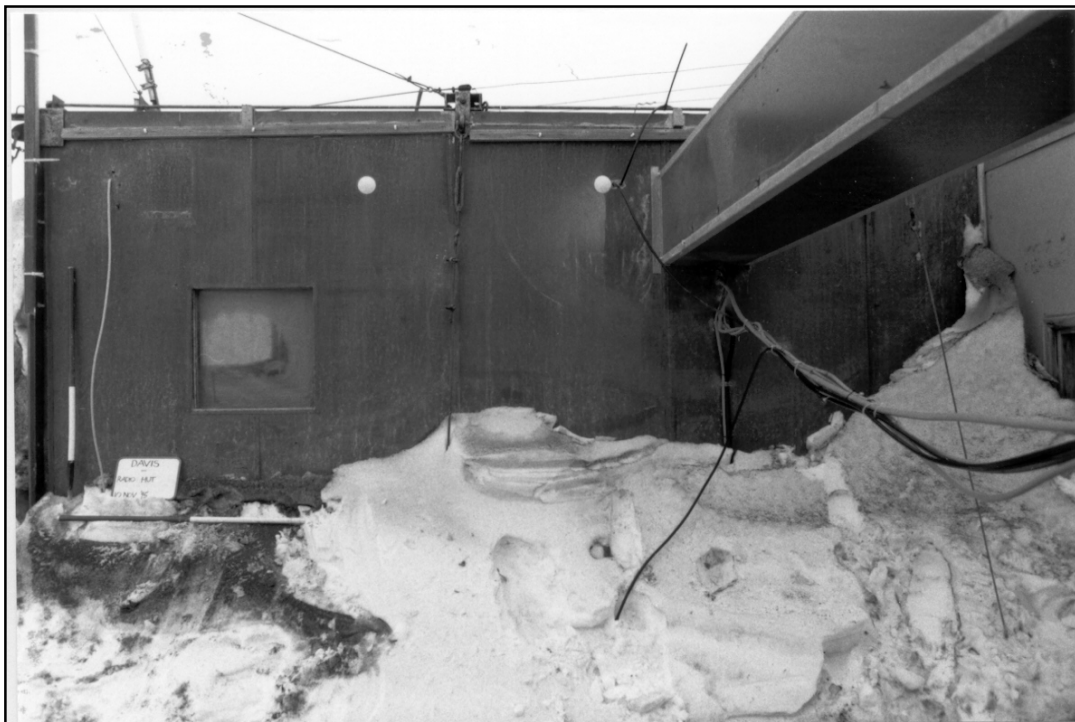
Radio Hut (View of southern side)
