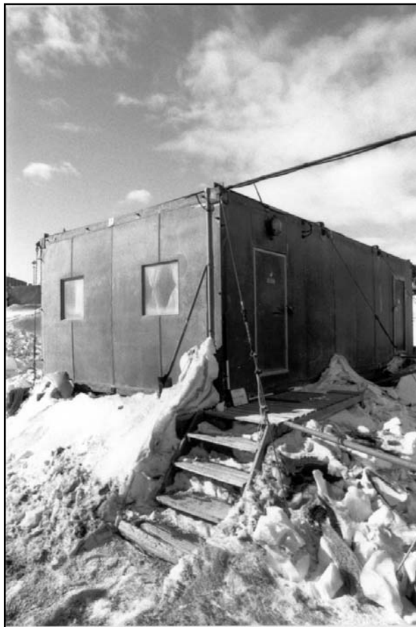
No.3 Store (View of southeast corner)
