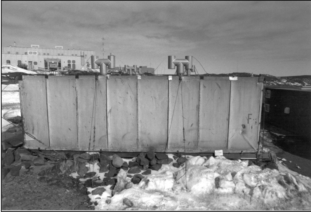
No.3 Store (View of northern side)
