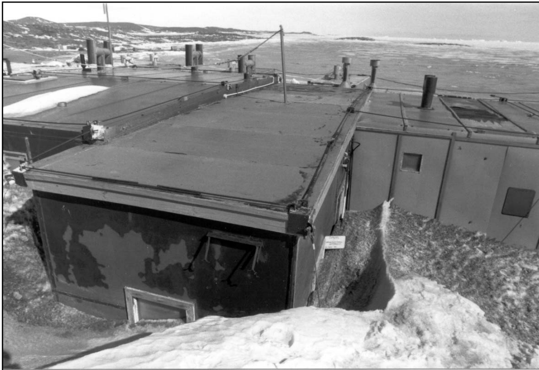
Office/Cold Porch/Bathroom (Viewed from the east)
