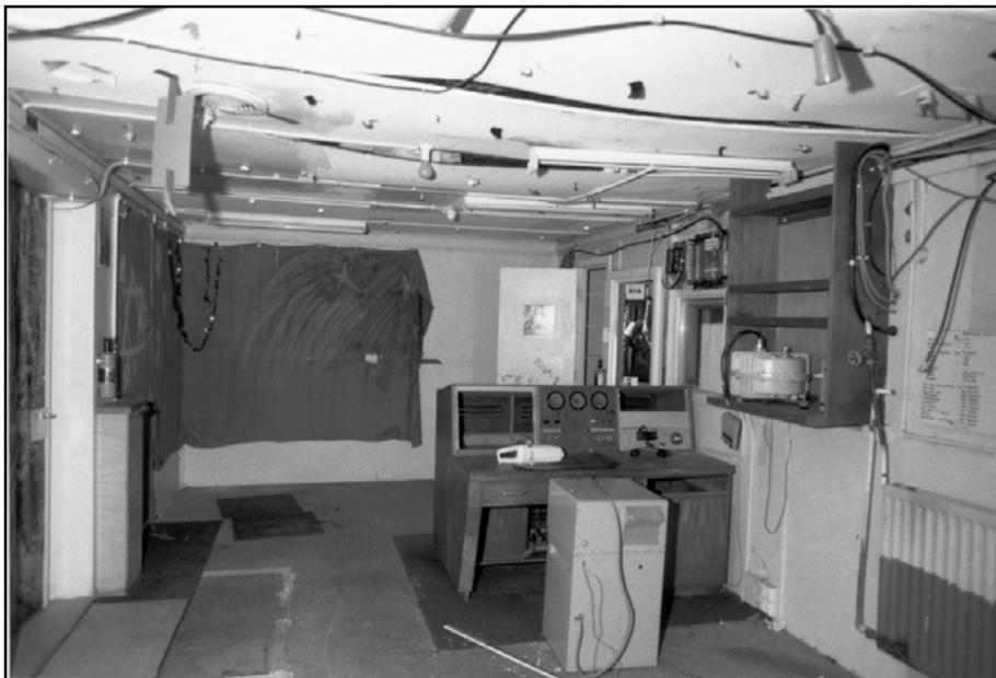
Radio Hut (Interior view looking east)
