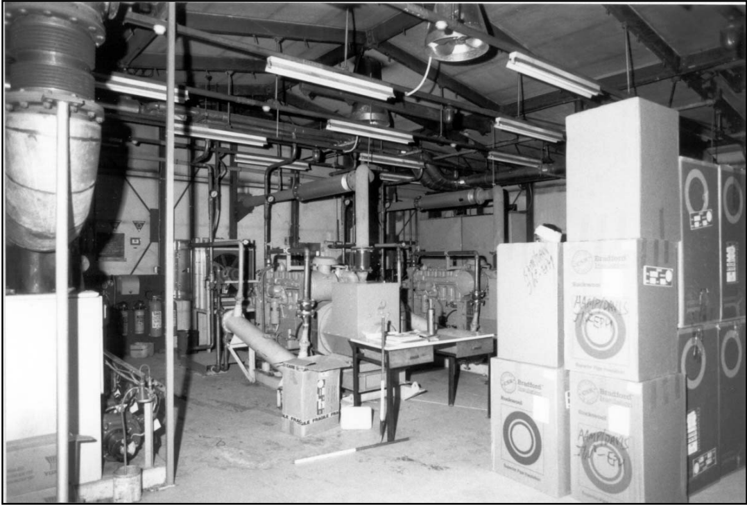
Emergency Powerhouse (Interior view)
