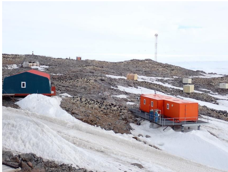
Figure 17. Scientific facilities, including cosmic radiation laboratory (front left), atmospheric laboratory (front right) and facilities for magnetic measurements (right mid-ground)
