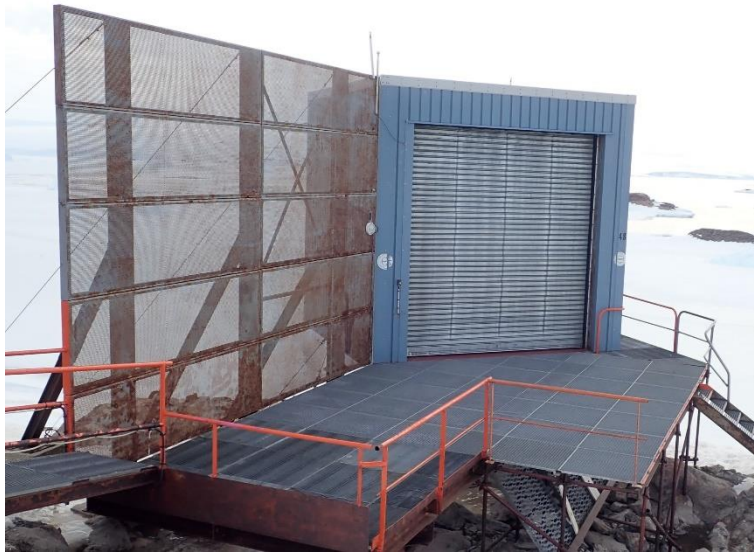
Figure 18. Meteorological balloon launching building
