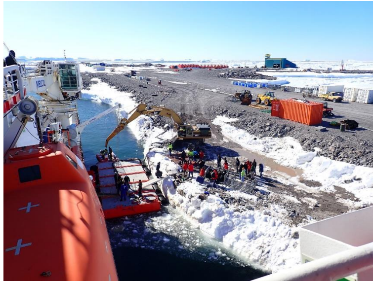
Figure 50. Unloading operations supported by ship crane, excavator and floating wharf
