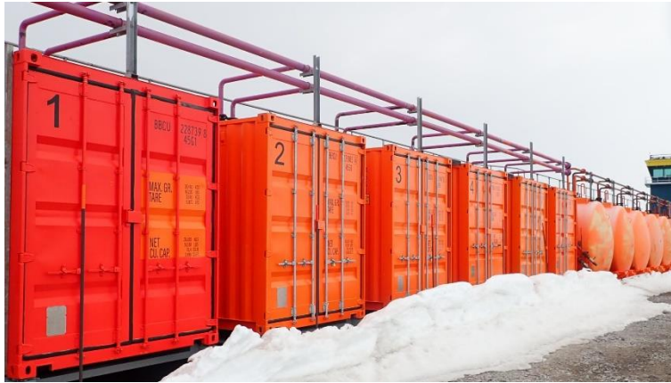
Figure 11. Bulk fuel storage tanks on Lion Island
