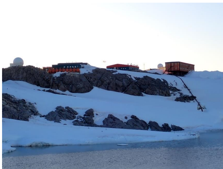
Figure 28. Waste water outlet from winter dormitory in upper station area
