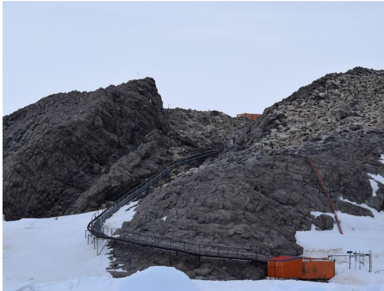
Figure 6. Elevated walkway from the east coast of Petrel Island to the upper station area
