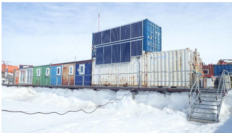
Figure 40. Solar panels on exterior of main station building
