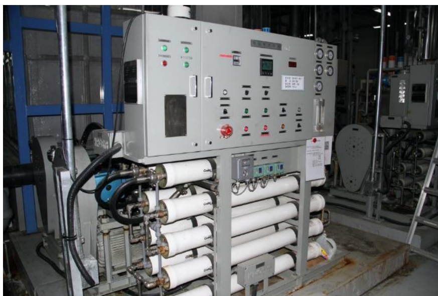
Photo: Reverse osmosis desalination equipment
