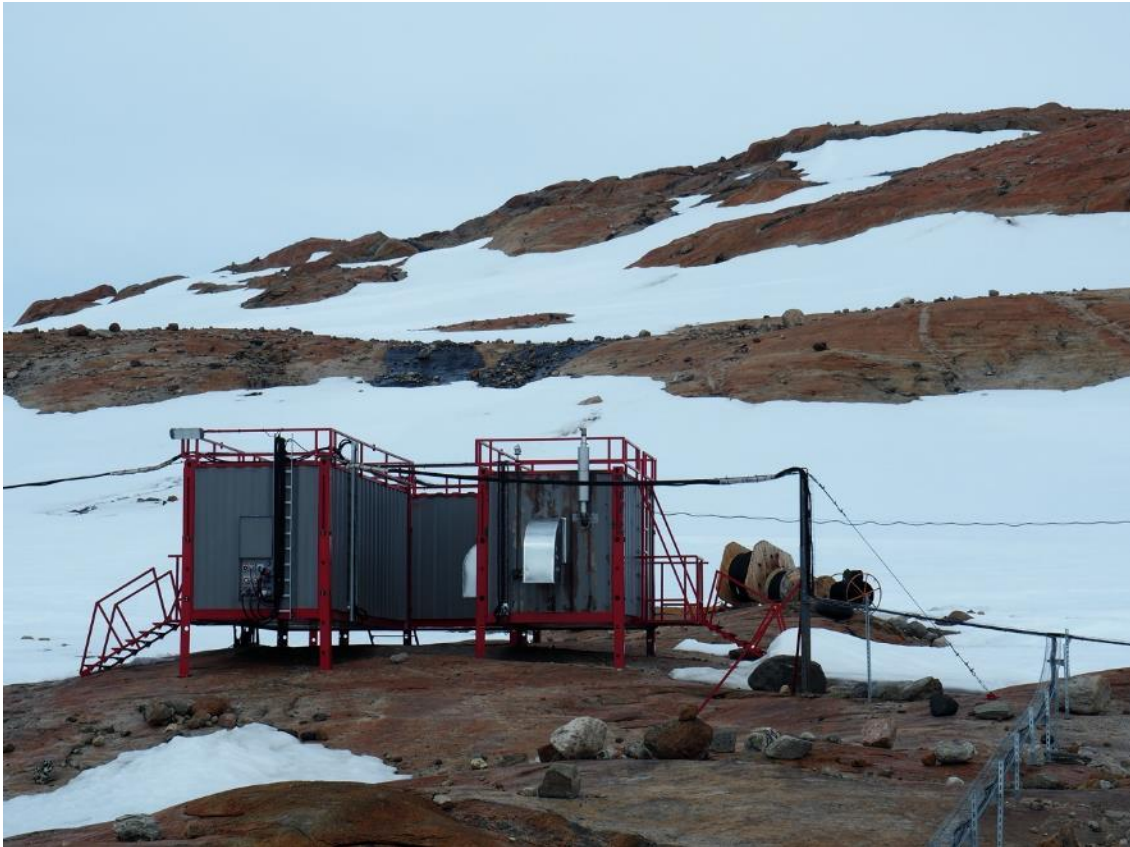
Photo: Containers housing diesel generators
