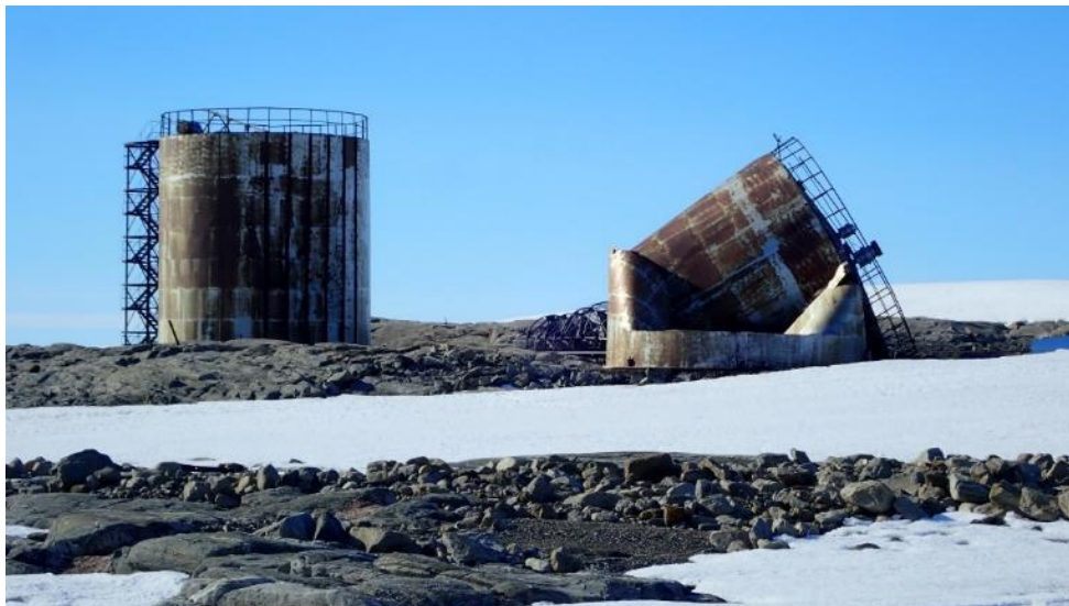
Photo: Damaged large fuel storage
