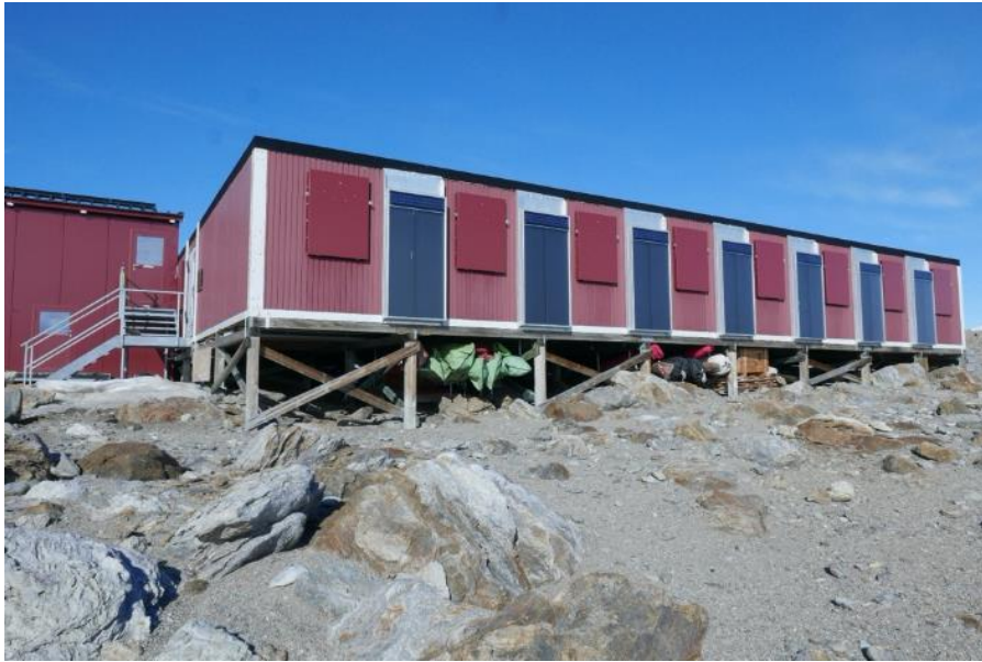
Photo: Solar thermal air heating panels on main building
