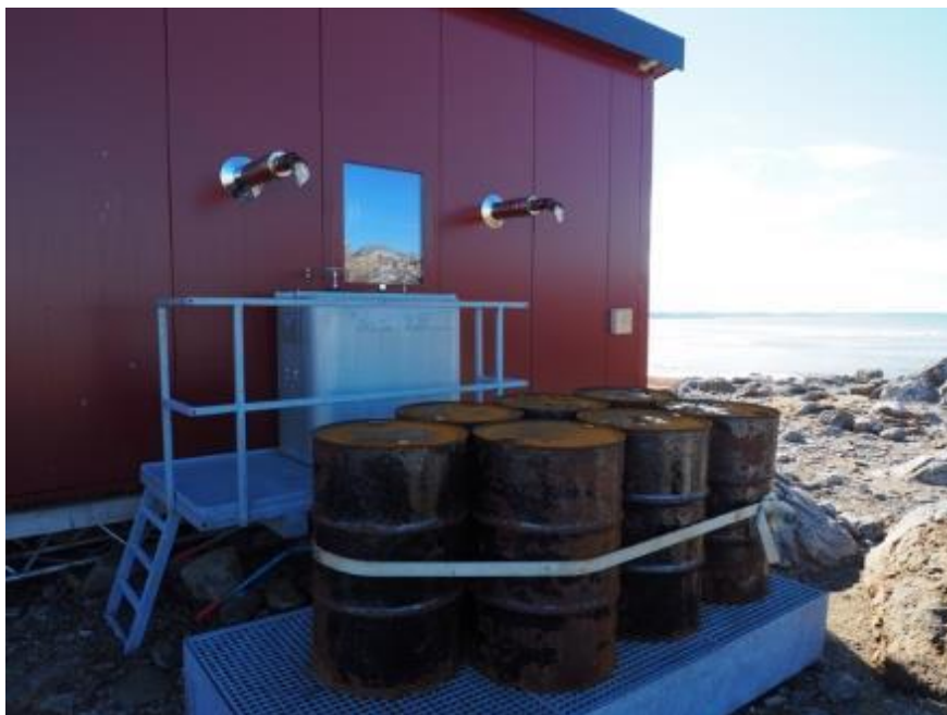
Photo: External fuel tank on power building, and drums on spill containment pallet
