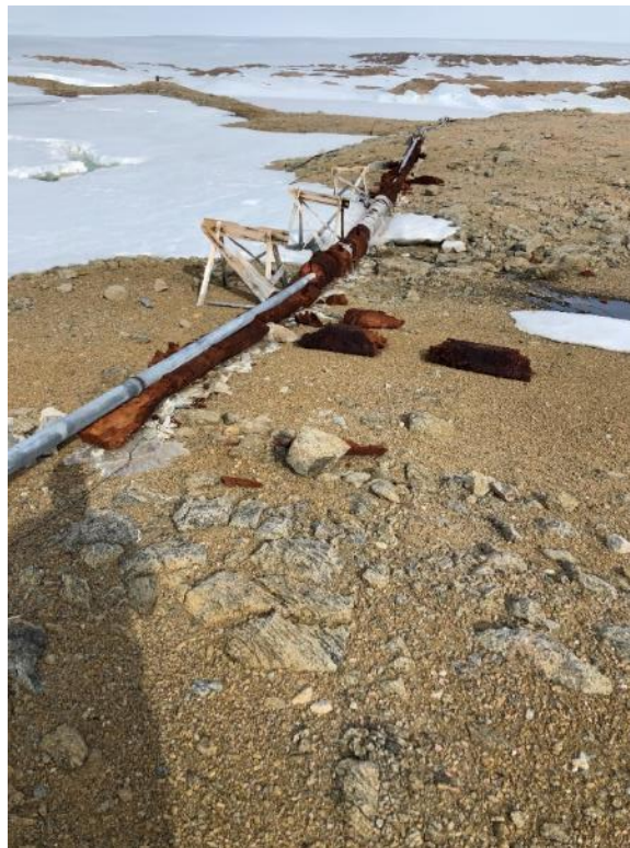
Photo: Water pipeline with deteriorated and liberated insulation
