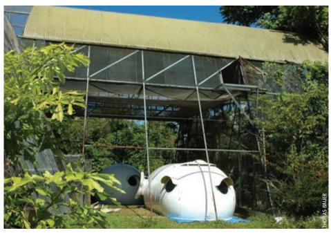
These extended 'tropicalised' Igloos, with tinted windows, window shade hoods and extended roof sections were originally used by the navy for hydrographic surveys on atolls off Far North Queensland. They are now in use at a Queensland resort.
