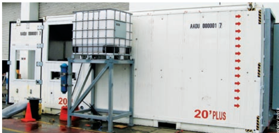
The containerised aquarium squeezes plant into one quarter of the total available space (behind the open door at left) and includes a separate seawater tank on a stand, to top up water levels.
