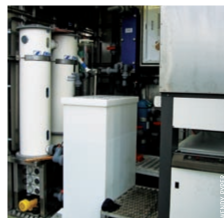
The aquarium plant includes a biological filter and degassing unit (white cylinders at left), a sump to distribute wastewater from the tanks to the various filters (white box at centre) and a chiller (bottom right) containing antifreeze used in the heat exchanger.
