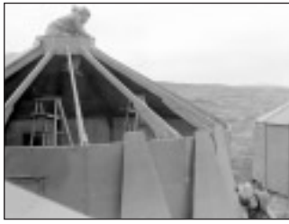
1948 Construction of 14-sided 5.6m diameter huts for radio/meteorological hut. These buildings were to prove technically successful but they are reported as having a rather depressing atmosphere.
