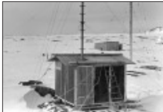
1948 Borden RAAF hut clad in masonite prefabricated panel construction, uninsulated, designed for the tropics. One of these buildings remains at Atlas Cove in 2001. The tractor garage can be seen over the top of the Dynes hut.
