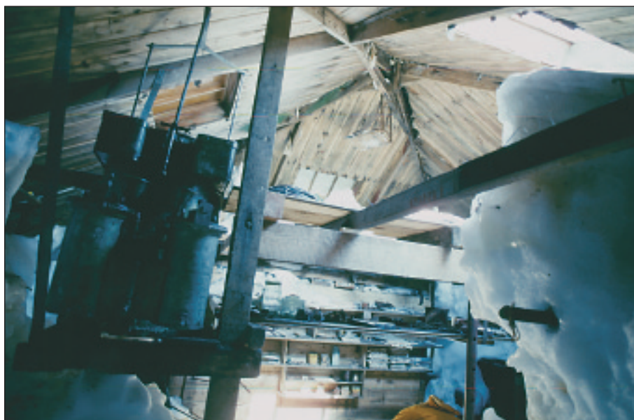
Interior of the main hut showing ice accumulation surrounding bunks and storage platform. In the left foreground is the acetylene plant used for lighting. ROB EASTER
