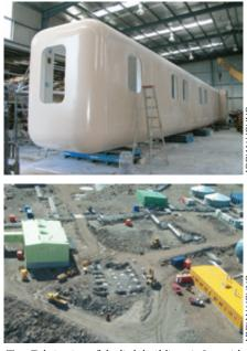
Top: Fabrication of the link building, 2.6 m wide x 3.4 m high x 23 m long, nears completion. Above: Aerial view of construction site with existing green living quarters at left, January 2004.
