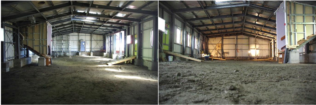
Figure 19. Current condition of the Old Living Quarters (internal) (Photo credit: Unknown)
