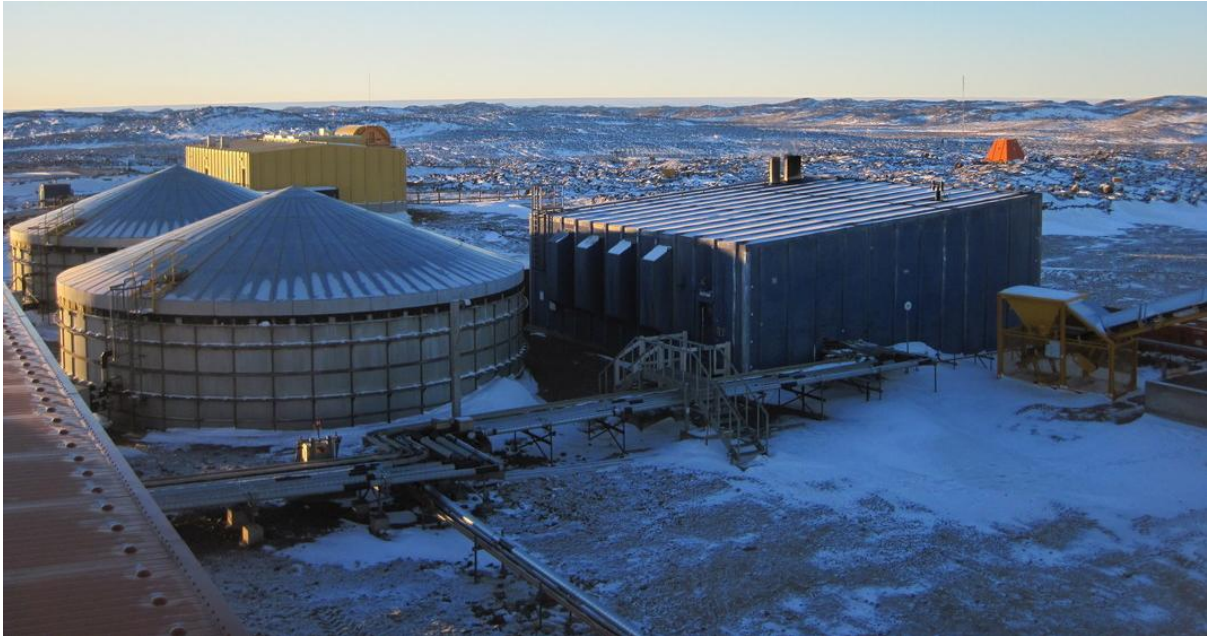
Figure 20. Davis station existing Main Powerhouse (blue) (Photo credit: Chris Hill)
