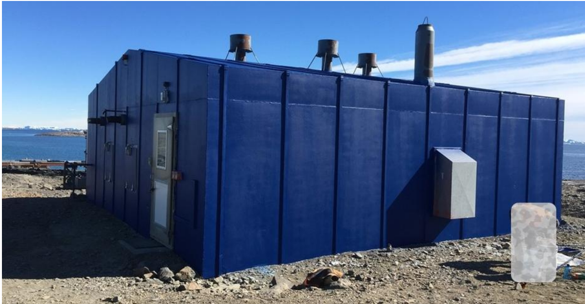
Figure 21. Davis station existing Emergency Powerhouse (Photo credit: Mark Booth)
