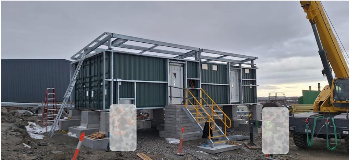
Figure 24. Davis station RO#1 during construction (2024–25) (Photo credit: Thomas De Leon)
