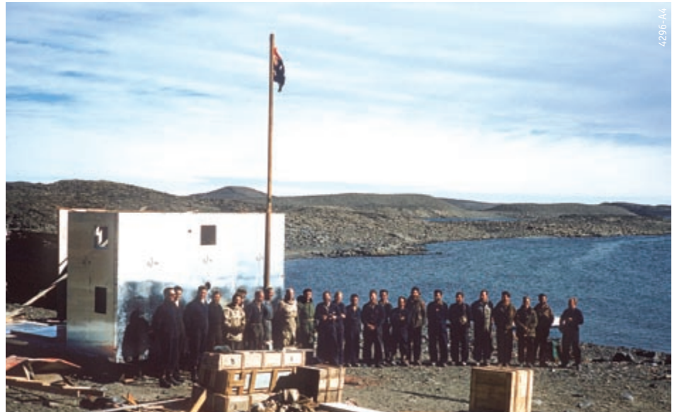
At 1600 hours on January 13th 1957, work stopped and all hands assembled around a flagpole, which had been strapped to the wall of the first hut being erected. Phil Law made a short speech stressing the importance of the new station in the International Geophysical Year programme. This was followed by short account of achievements of Captain John King Davis, the singing of God Save the Queen, three cheers, and then back to work.
