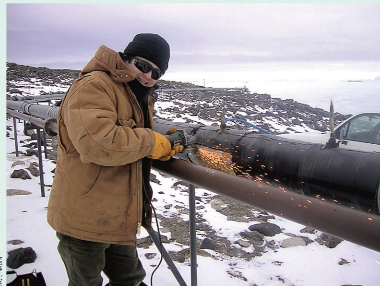
Cutting the sewage line in order to clear a blockage.
