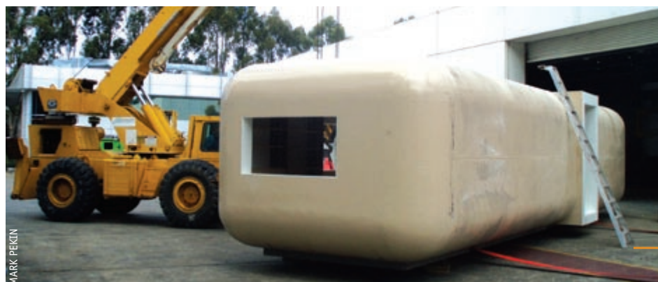
The prefabricated fibre composite building weighs about seven tonnes.
