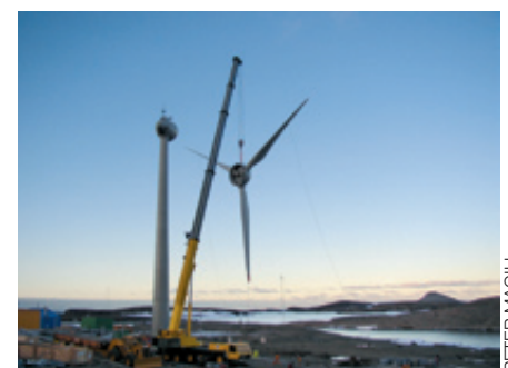
From top: The new Mawson skyline; towing the bottom tower section to the turbine site; lifting the hub and blade assembly onto the turbine nacelle.
