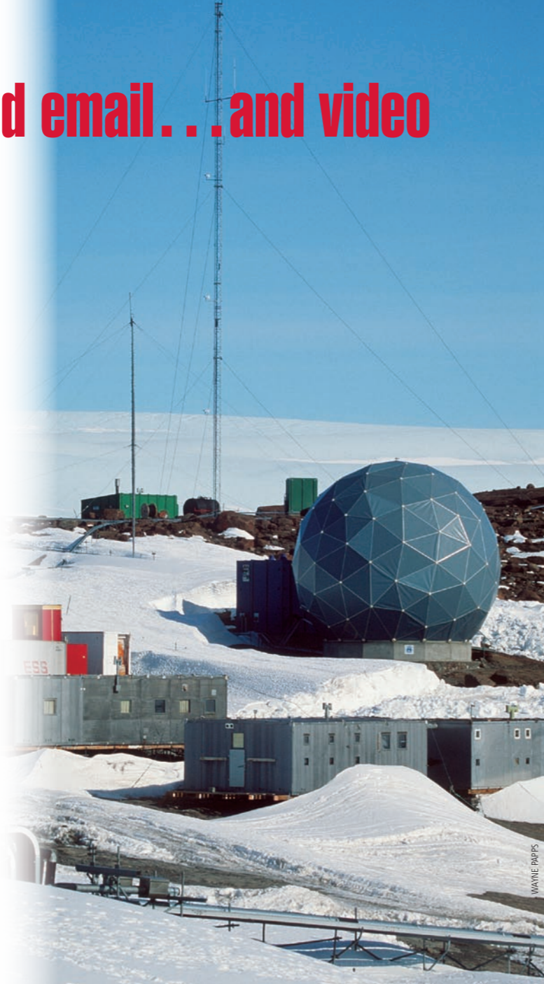
The Mawson ANARESAT radome was commissioned in January 1988. This satellite network infrastructure, established on each of Australia's stations, allows expeditioners to use satellite-based phone, email, internet and fax services to communicate with Australia. Radio masts can be seen in the background.
