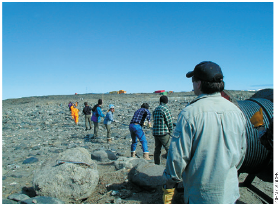
Davis expeditioners help roll out the power cable for the VHF radar installation.
