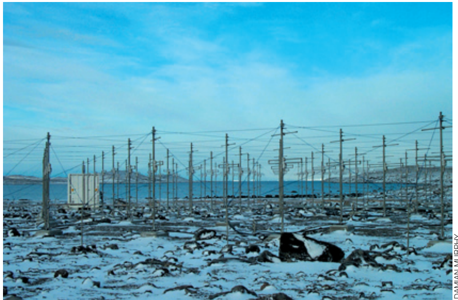
VHF radar antennas after installation at Davis
